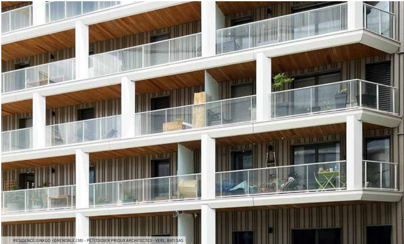
RESIDENCE GINKGO - GRENOBLE (38) - PETITDIDIER PRIOUX ARCHITECTES - VERL. BATI SAS
