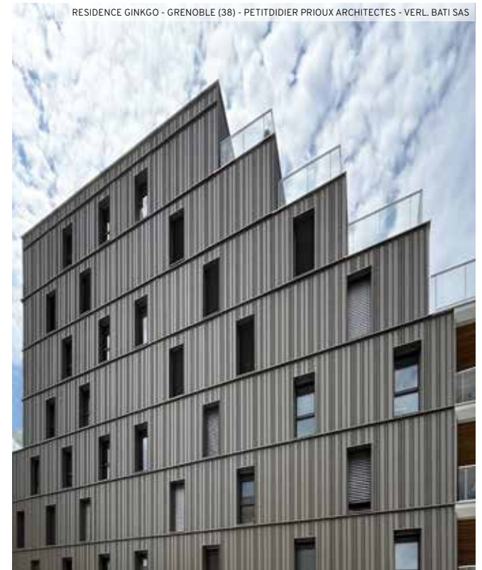
RESIDENCE GINKGO - GRENOBLE (38) - PETITDIDIER PRIOUX ARCHITECTES - VERL. BATI SAS
