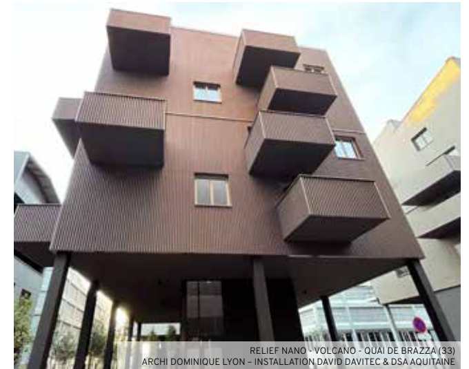
RELIEF NANO - VOLCANO - QUAI DE BRAZZA (33) ARCHI DOMINIQUE LYON - INSTALLATION DAVID DAVITEC & DSA AQUITAINE
