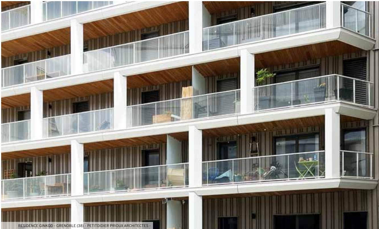
RESIDENCE GINKGO - GRENOBLE (38) - PETITDIDIER PRIOUX ARCHITECTES -
