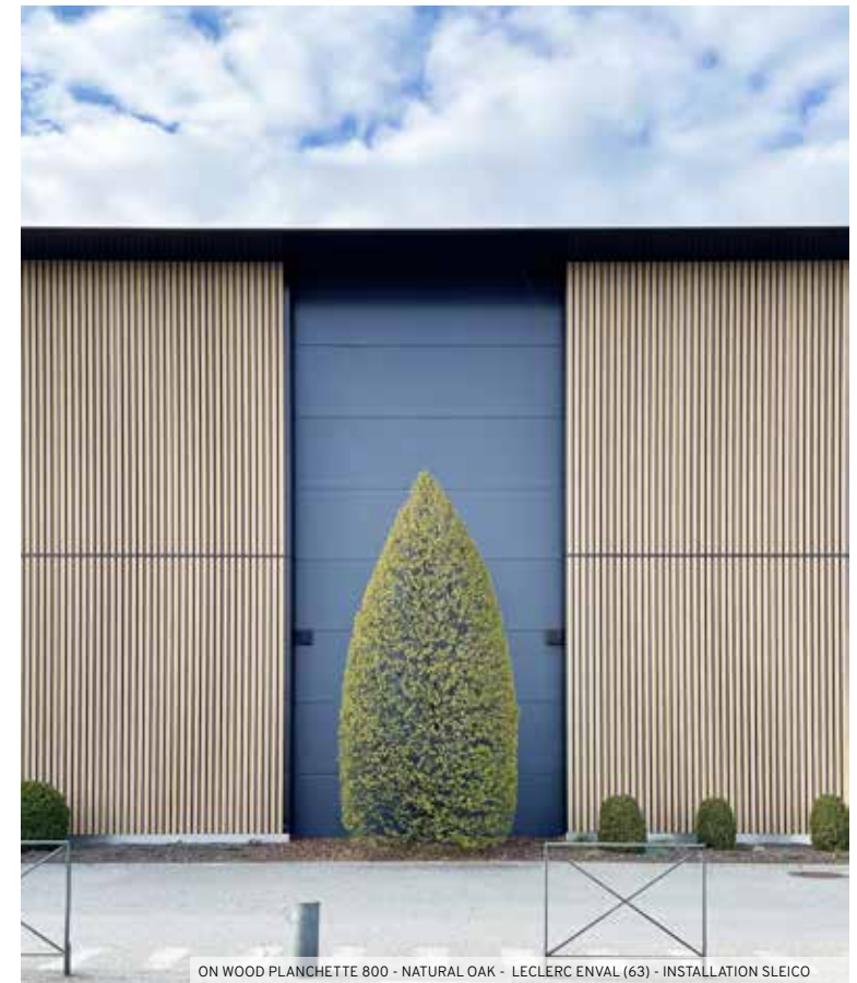
ON WOOD PLANCHETTE 800 - NATURAL OAK - LECLERC ENVAL (63) - INSTALLATION SLEICO
