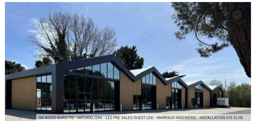
ON WOOD BARO 710 - NATURAL OAK - LES PRE SALES OUEST (33) - MARRAUD INGENIERIE - INSTALLATION STE ELIXE
