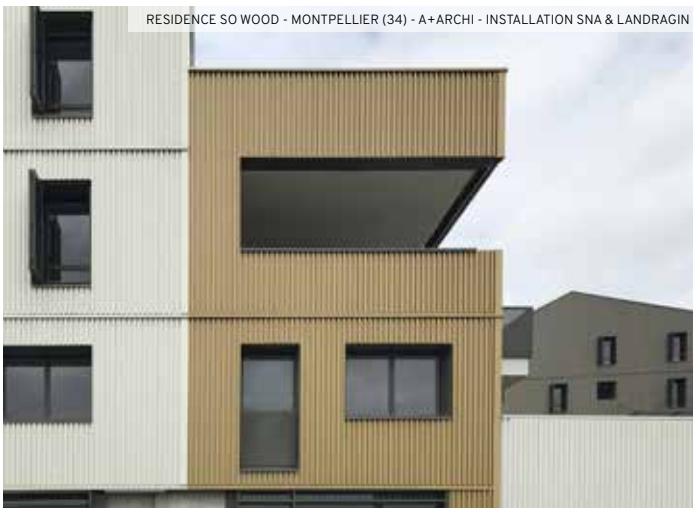
RESIDENCE SO WOOD - MONTPELLIER (34) - A+ARCHI - INSTALLATION SNA & LANDRAGIN
